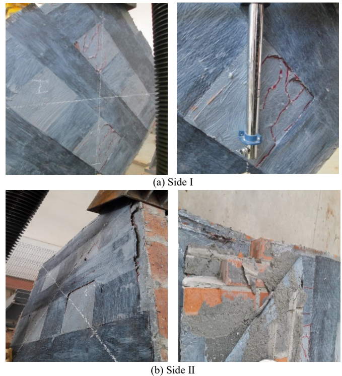
Figure 7: Diagonal shear cracking along the diagonal and delamination of CFRP wraps of the strengthened wall
