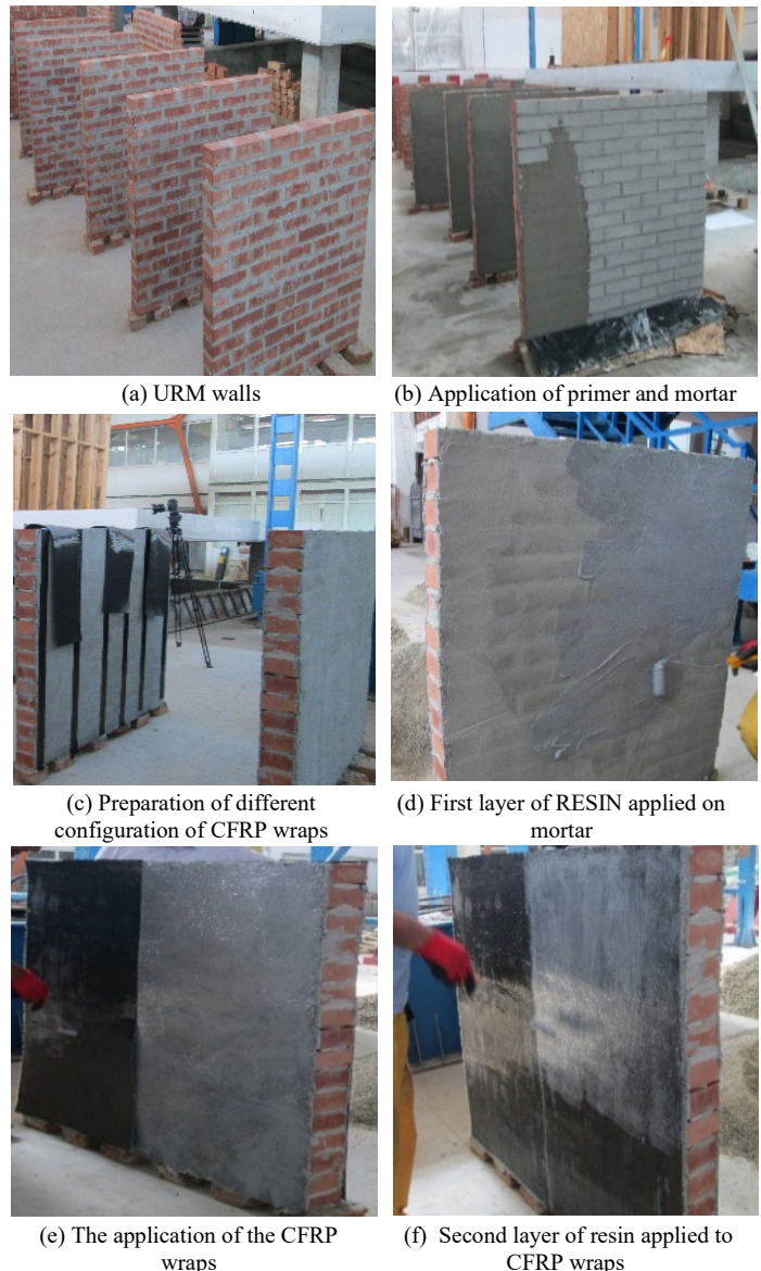
Figure 1: Different steps of retrofitting URM wall by the CFRP wraps
