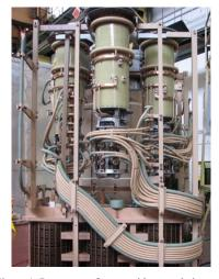
Figure 1: Power transformer with a regulation unit
