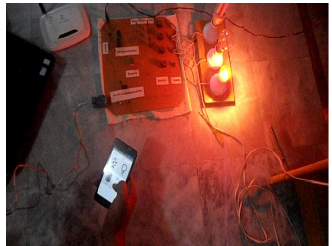
Figure 12: Complete System in Working
