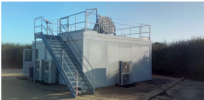
Fig.3. Transmitting system (the shelters with the antenna on the roof without the radome)
