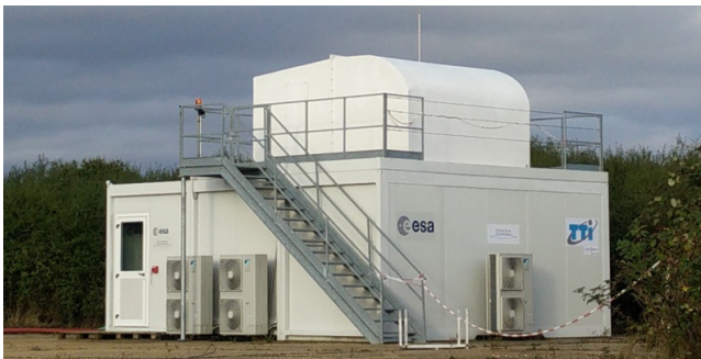
Fig.2. The transmitting system the shelters with the antenna on the roof (under a radome)
